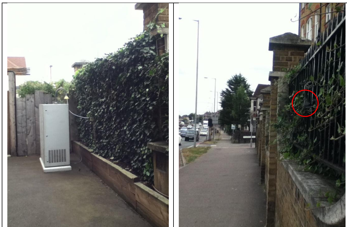
Figure 5: Monitoring station and inlets situated on the playground side of the green screen (left) and the roadside of the screen (right)
