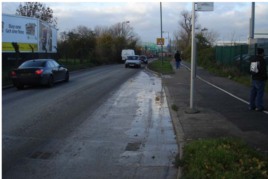
Figure 6 Substantial silting in a bus stop on Beddington Lane to the south of Country Waste Management Ltd.
